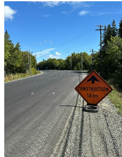
Highway 105 – September 2025, Repaving 100-Series Highways (Office of the Auditor General photo)
