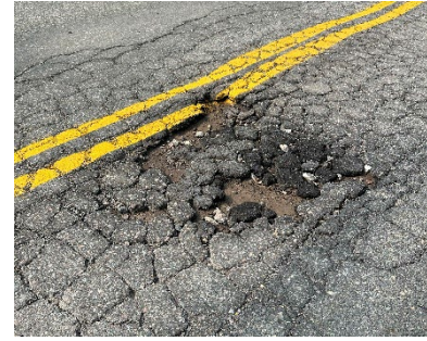
Local Road – Pothole and Alligator Cracking, September 2025 (Office of the Auditor General photo)
